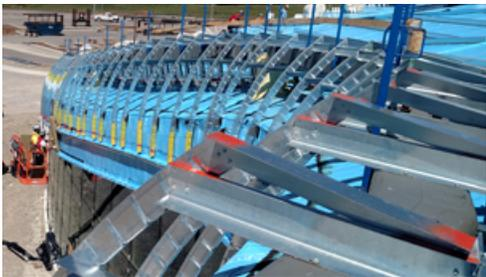
Pre-curved trusses set parapet geometry of the
