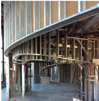
Pre-fabricated Curved-Right® and hand-bendable Ready Product combine to create curved and complex surfaces
